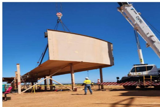
Boonanarring WCP Dismantling
